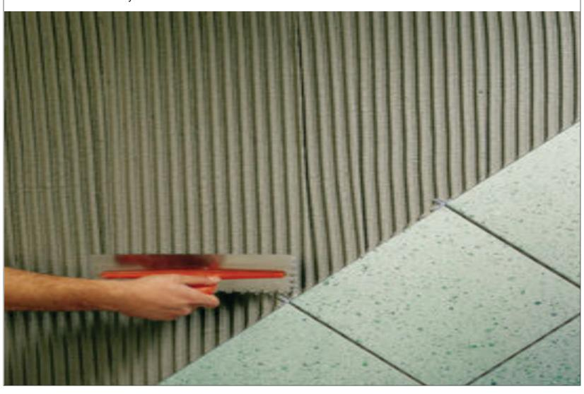
BCM 09 Premium Adhesive is a professional grade, polymer modified thin-set mortar for interior and exterior floor and wall applications of all types of ceramic tile, most types of porcelain tile and stone over most traditional and speciality substrates.
